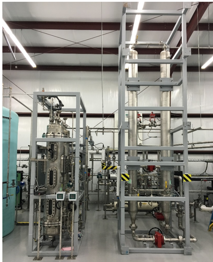
Fig. 6. Ion Exchange Columns (left) Cross Flow Filters (Right)
