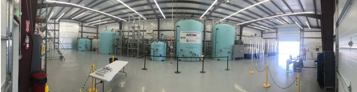
Fig. 5. Engineering Scale Test Rig Overview
